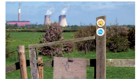
Cottam Power Station from Dunham.
